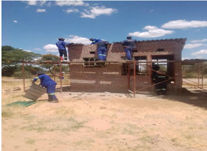
Roofing of a guardroom at Khami Agriculture by Carpentry Trainees
